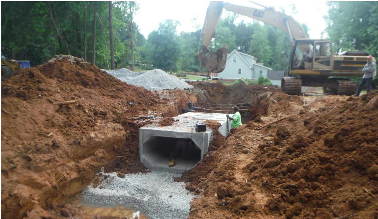
Photo 2: Installation of new box culvert sections.
