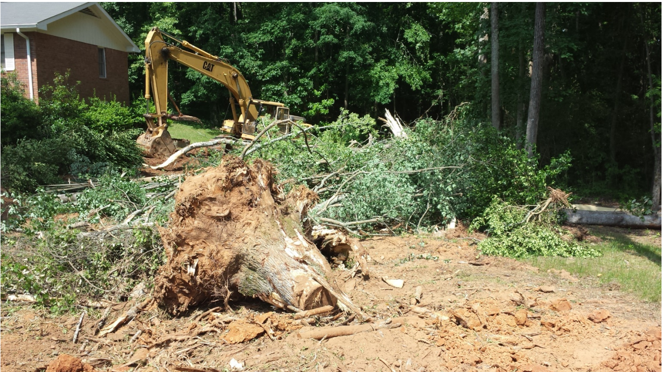
Photo 2: Clearing underway to provide proper area to redirect the stream for new culvert placement. (05/28/2014)
