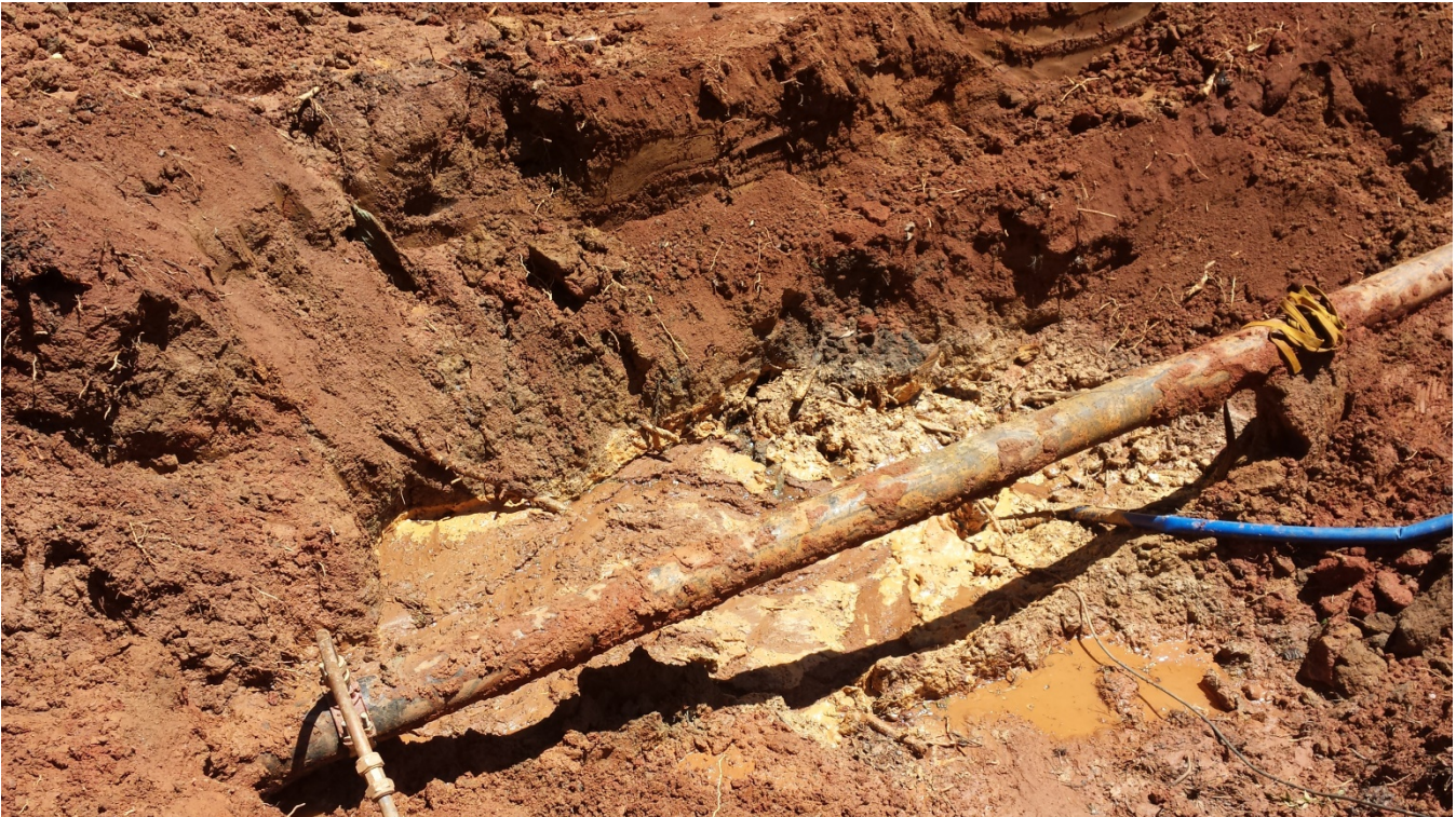
Photo 2: A water line at the project location exposed and ready for relocation, to allow for installation of new box culvert.
