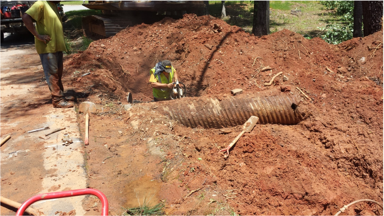
Photo 1: Construction underway to remove old pipe.
