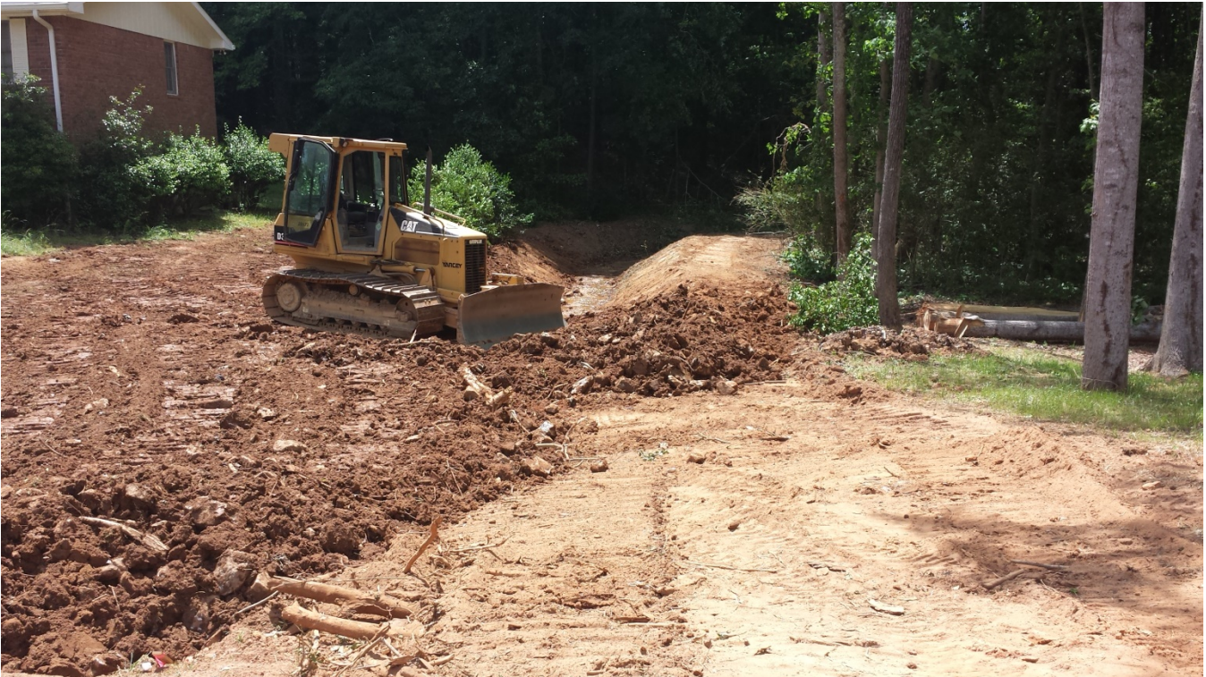
Photo 1: Clearing and grading continues for stream redirection. (05/29/2014)
