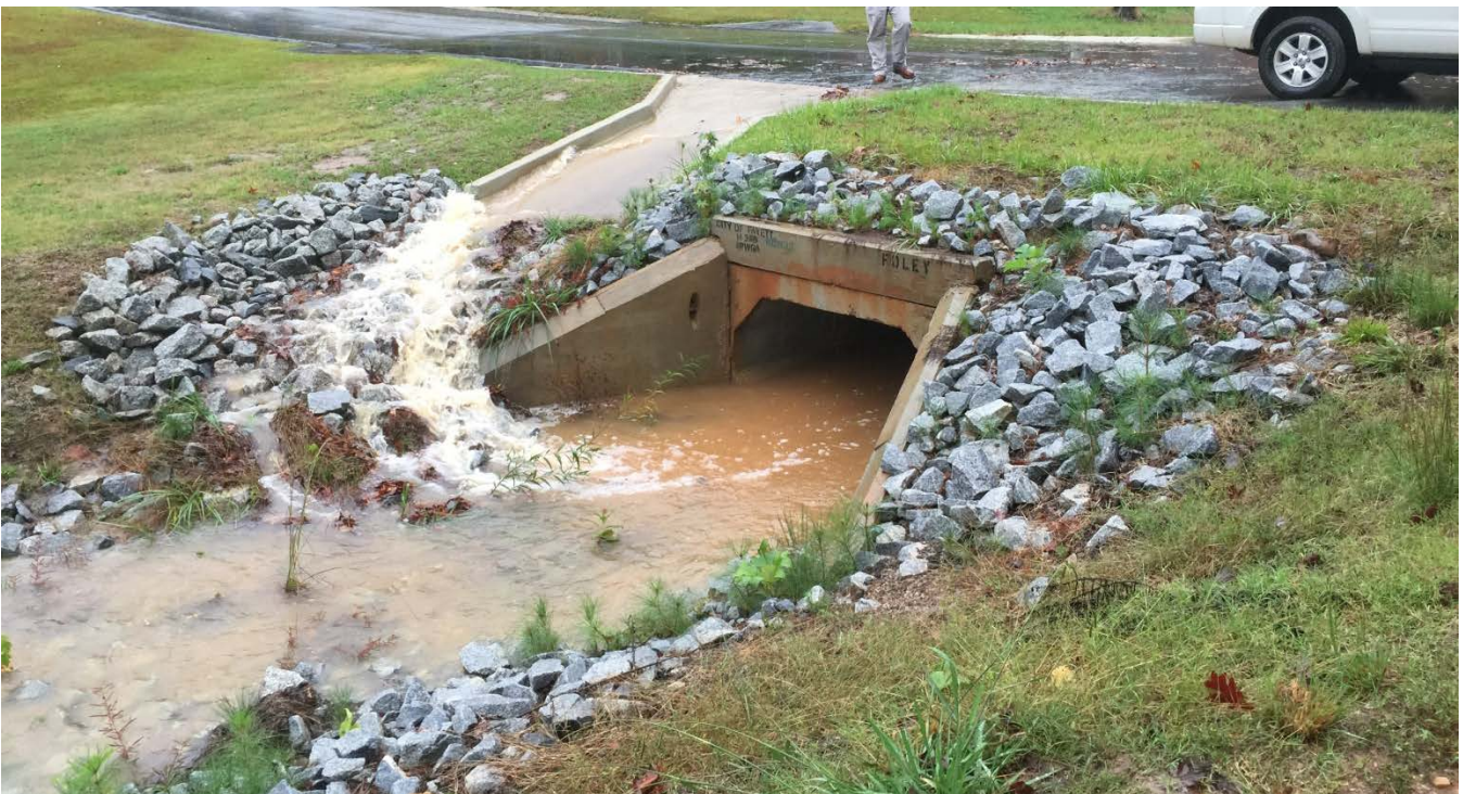
Photo 2: View of inlet side of new culvert. Rain event shows the culvert and curb and gutter operating successfully.
