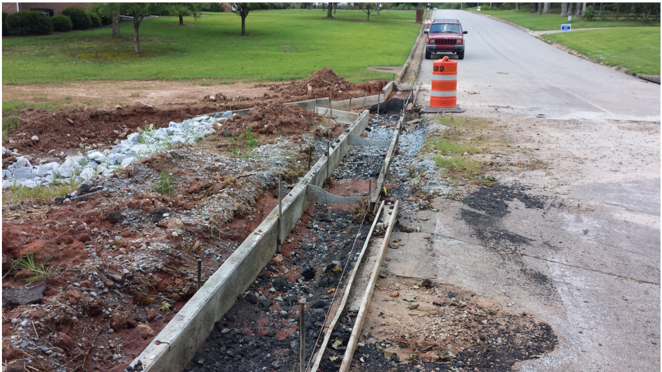
Photo 2: Curb and gutter are being framed to prep for concrete pouring. (08/21/2014)
