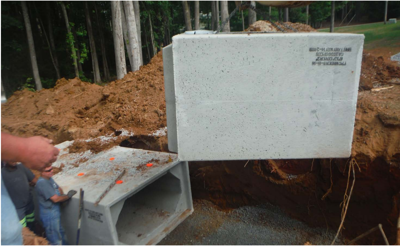
Photo 1: Installation of new box culvert sections.
