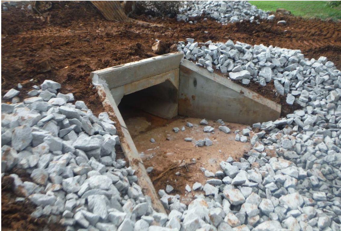
Photo 1: Installation of new headwall. (06/12/2014)
