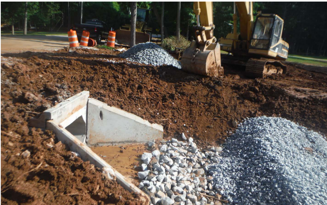
Photo 2: Grading work underway. (06/13/2014)
