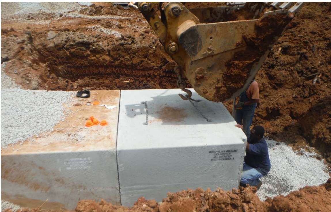
Photo 2: Installation of new box culvert sections. (06/04/2014)
