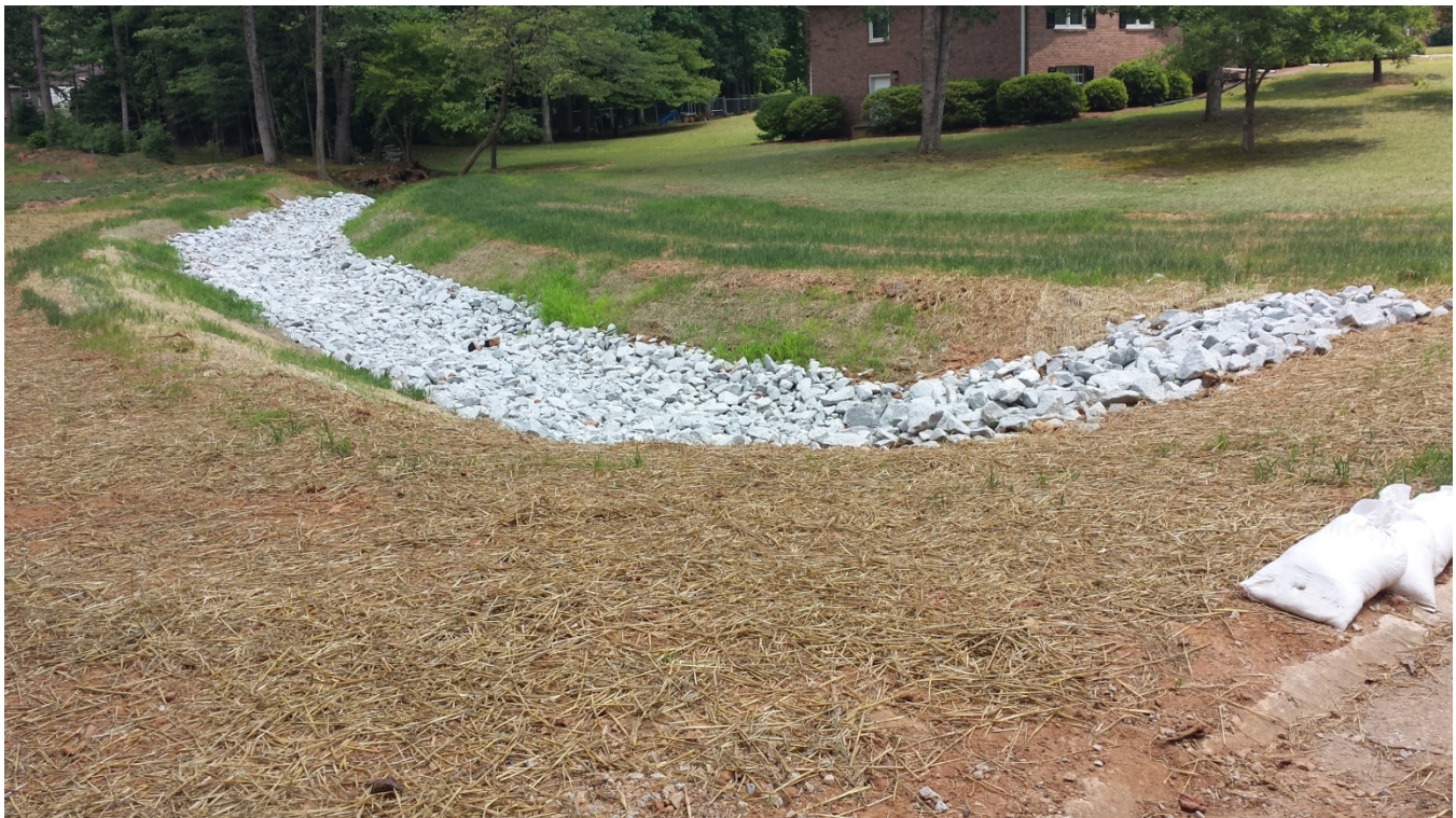
Photo 2: Grass is beginning to grow alongside the new culvert and stream. (07/08/2014)
