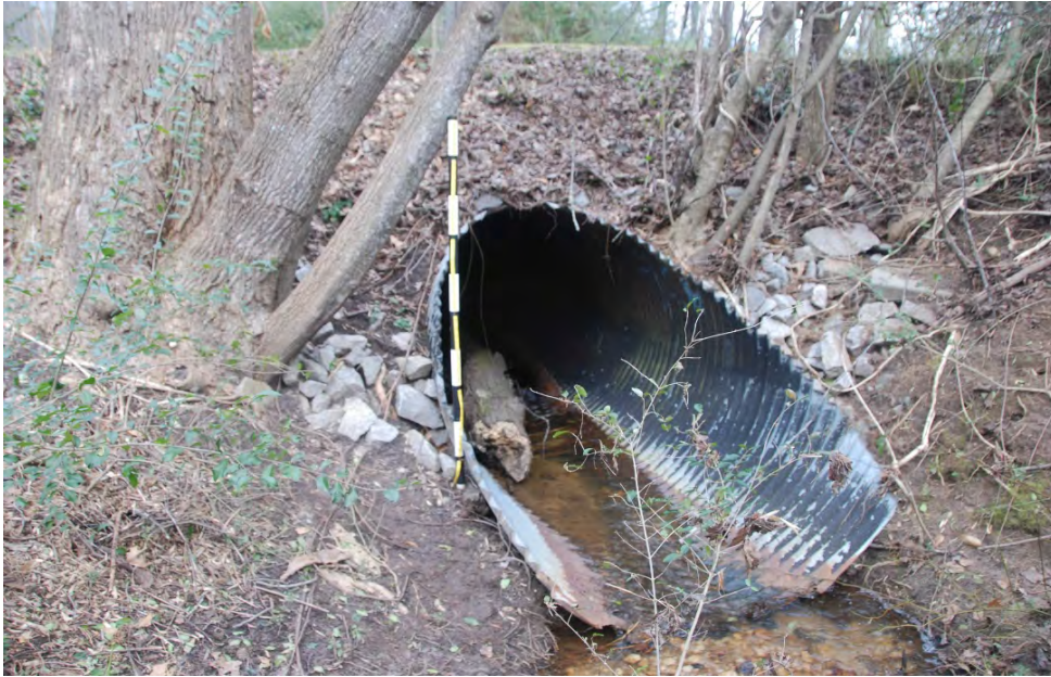
Photo 1: Upstream end of culvert.
