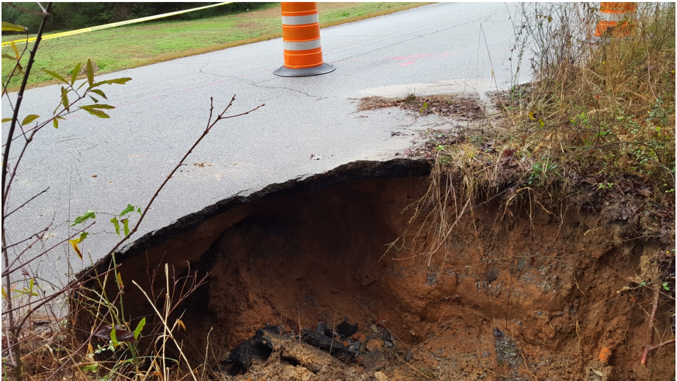
Photo 1: Pre-existing condition. During the December 2015 and New Year's (2016) rain events, two 36" metal pipes failed causing imminent road failure. This shows washout underneath road on downstream side of pipe.
