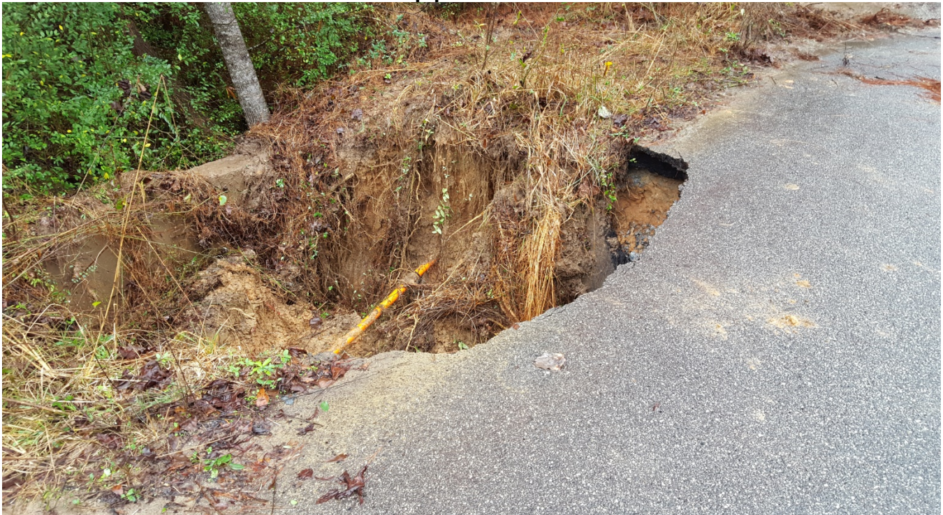
Photo 2: The shoulder of the road washed away exposing a gas line.
