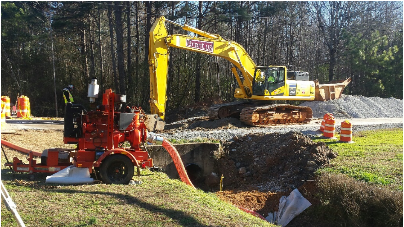
Photo 1: Excavation began at project location. The water was pumped around the location to provide dry site conditions.
