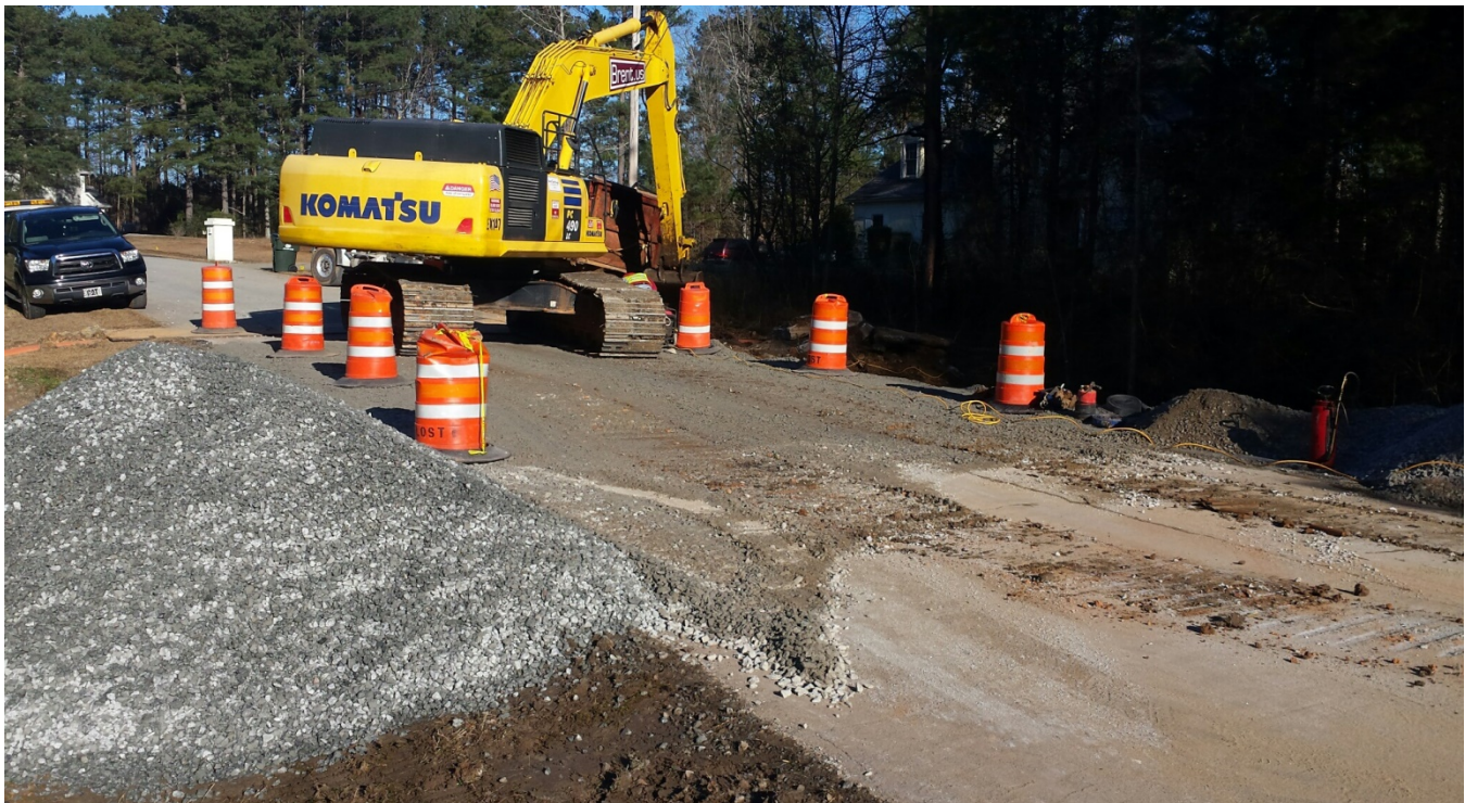
Photo 2: The roadway is prepared for paving.
