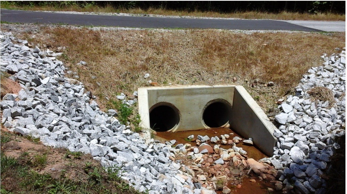
Photo 1: The two new 36" concrete pipes and headwalls have been installed. Rip rap was placed around the project area. (Work completed 01/14/2016)
