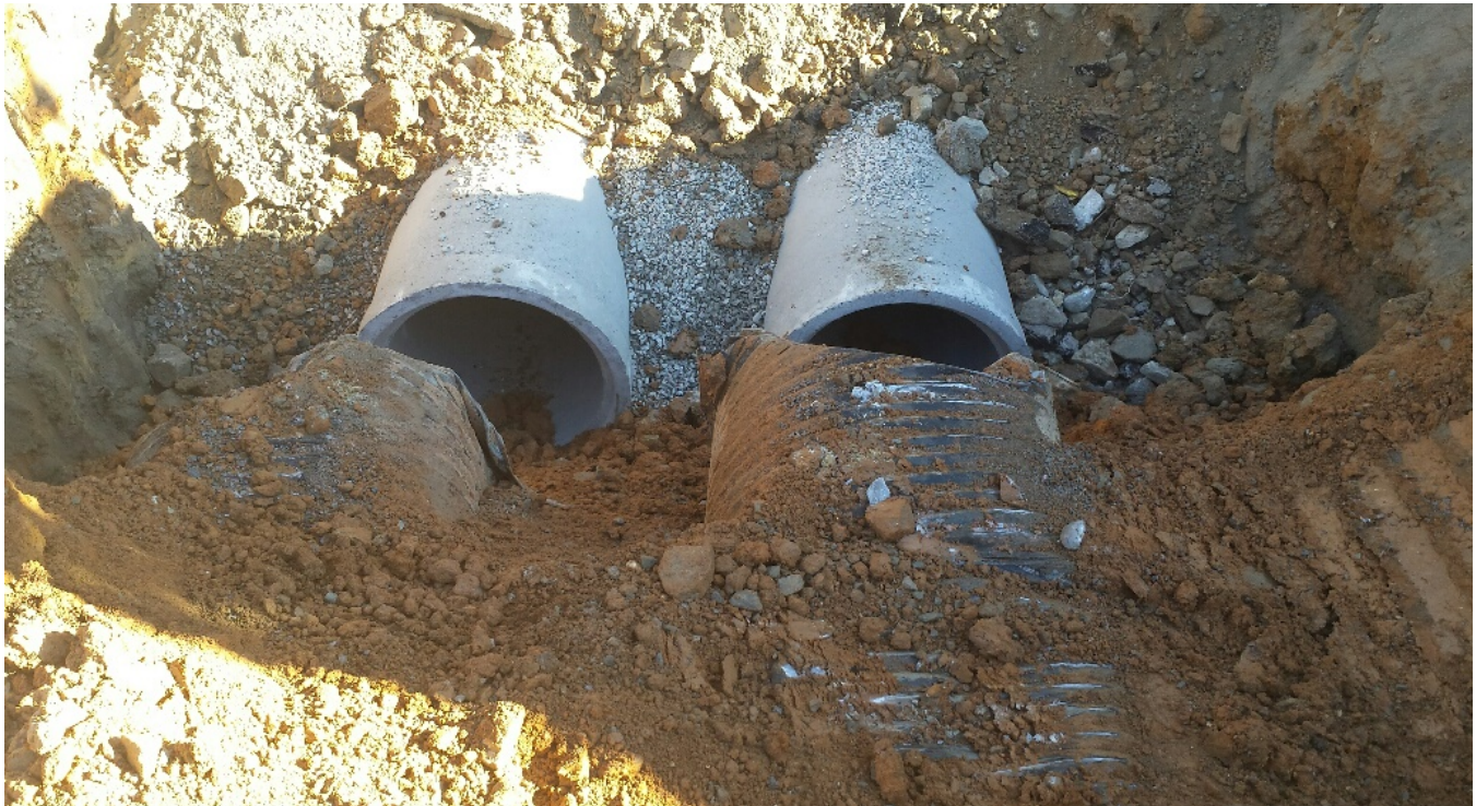
Photo 2: The existing pipes were removed and replaced by two 36" concrete pipes.
