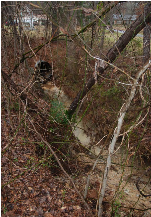
Photo 2: Downstream end of culvert looking east towards Ridge Way.
