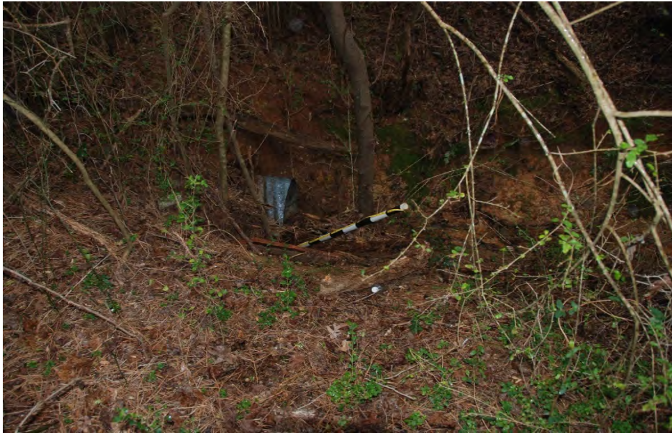
Photo 1: Upstream end of culvert.
