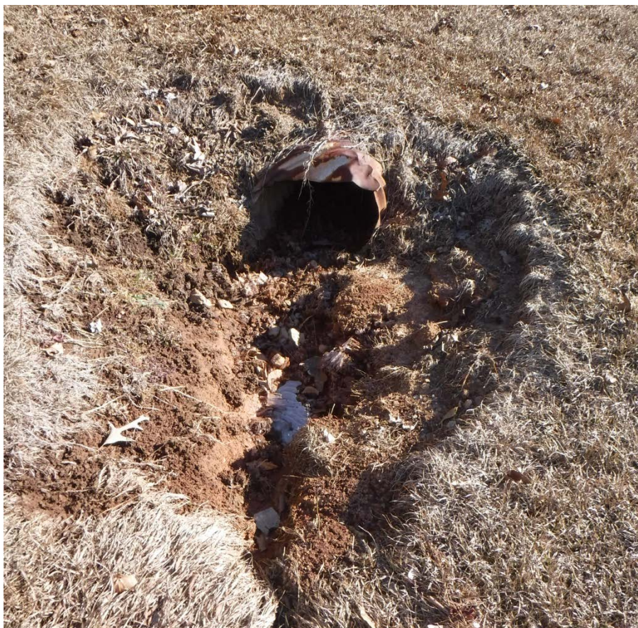
Photo 2: Pipe condition prior to replacement
