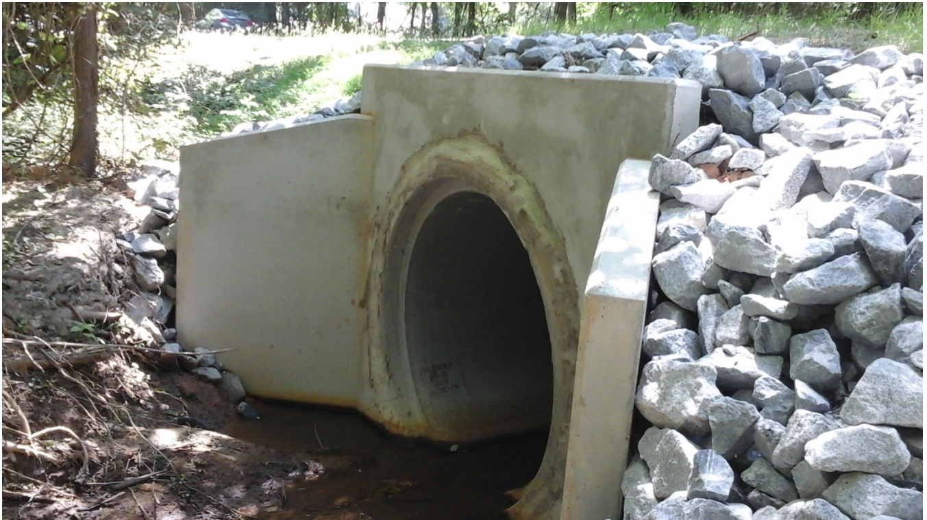
Photo 1: Completed project. Photo captures new headwall that was installed.
