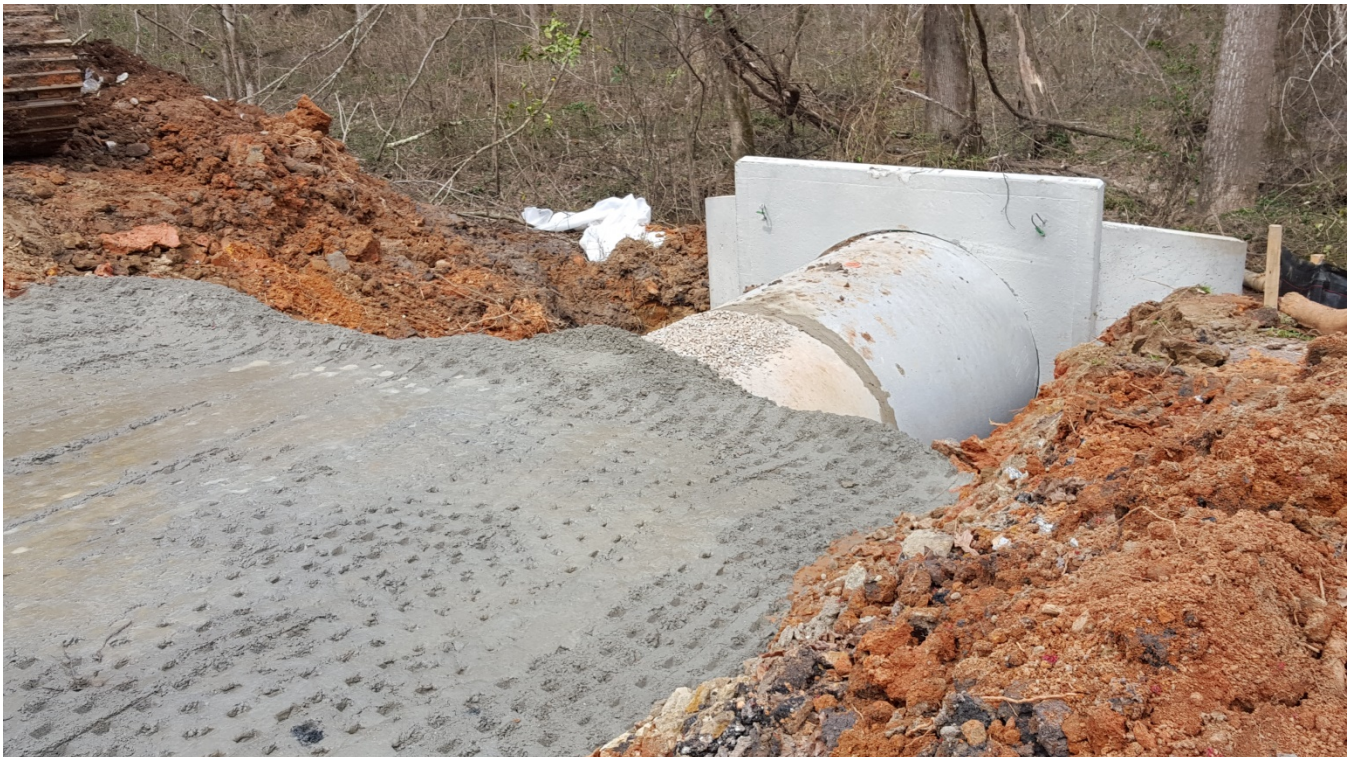
Photo 2: Installation of headwall and location grading. (03/08/2016)
