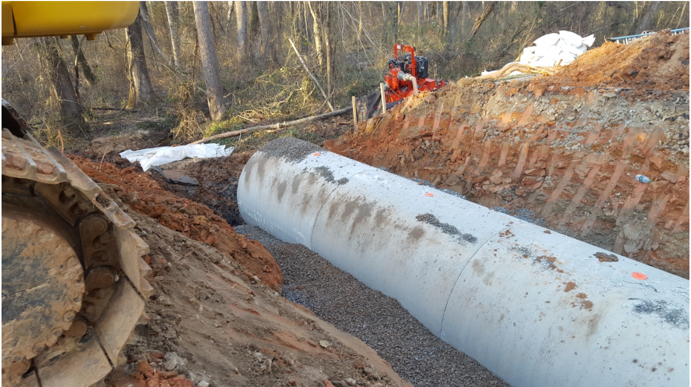
Photo 1: Installation of 42" concrete pipe. (03/07/2016)
