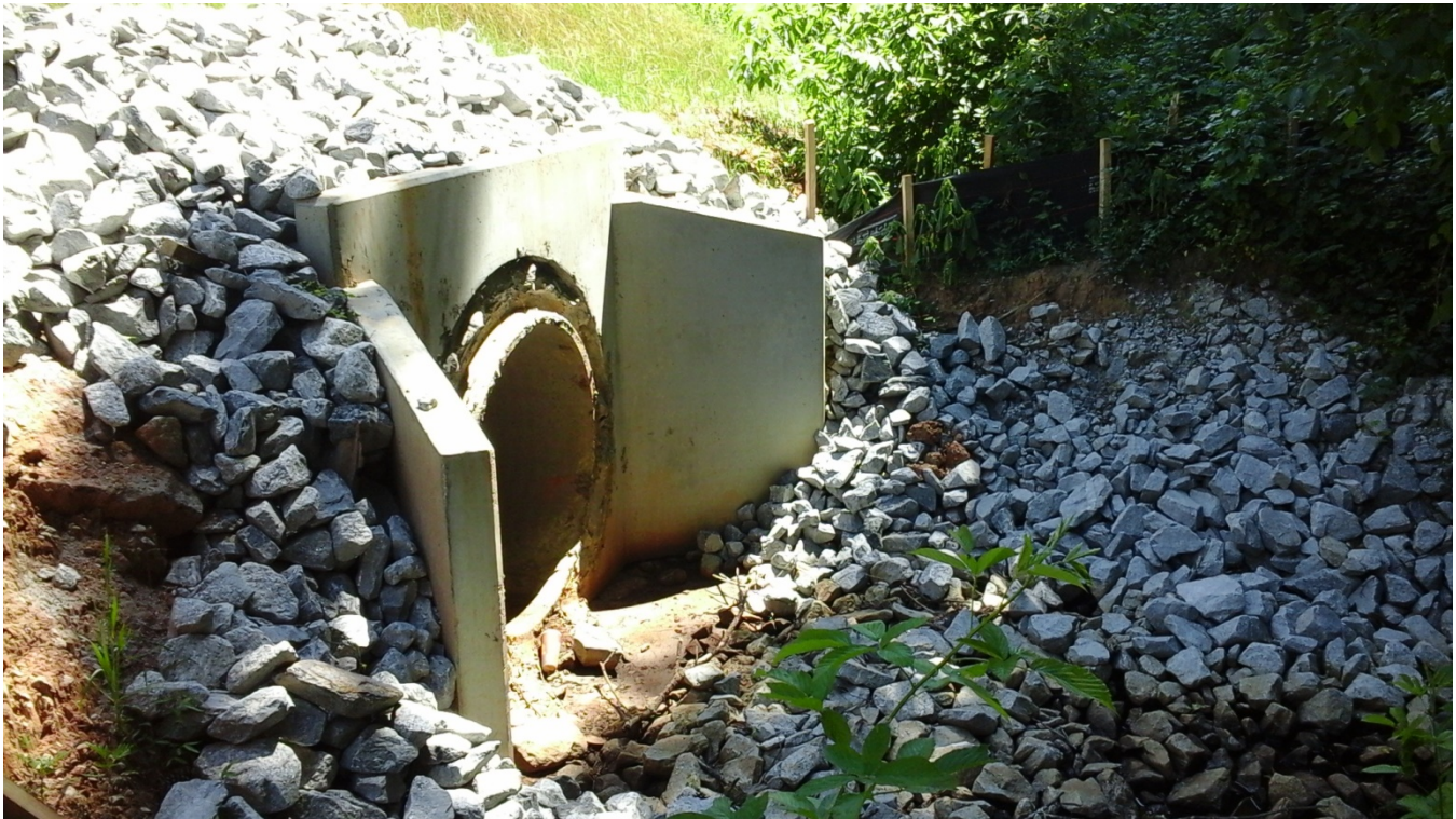
Photo 1: The new 54" concrete pipe and headwalls have been completely installed, along with rip rap along the shoulder and creek bed.
