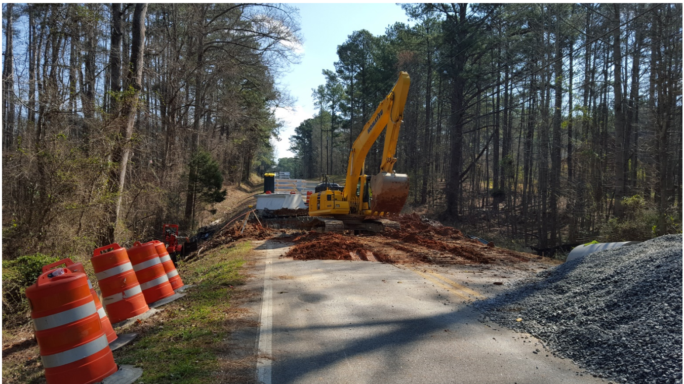
Photo 2: Excavation at the project location to remove excess materials and dirt to prepare for pipe installation.
