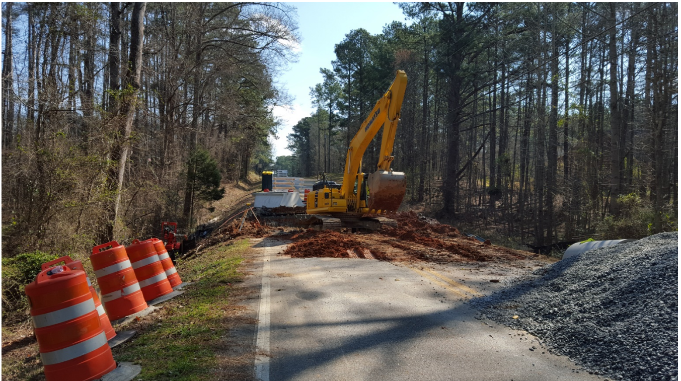
Photo 2: There was a large void between the washout pipe and the bottom of the road surface. The road was collapsed by the Road Department, to prevent vehicles from driving across the road resulting in catastrophic accidents until the pipe could be replaced.
