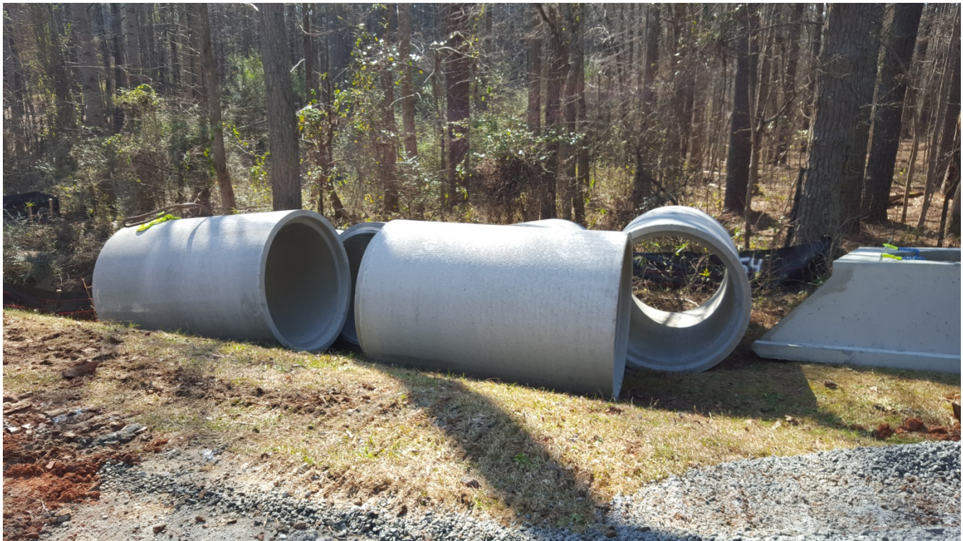
Photo 1: The new 54" concrete pipe and headwalls were delivered and staged until installation.
