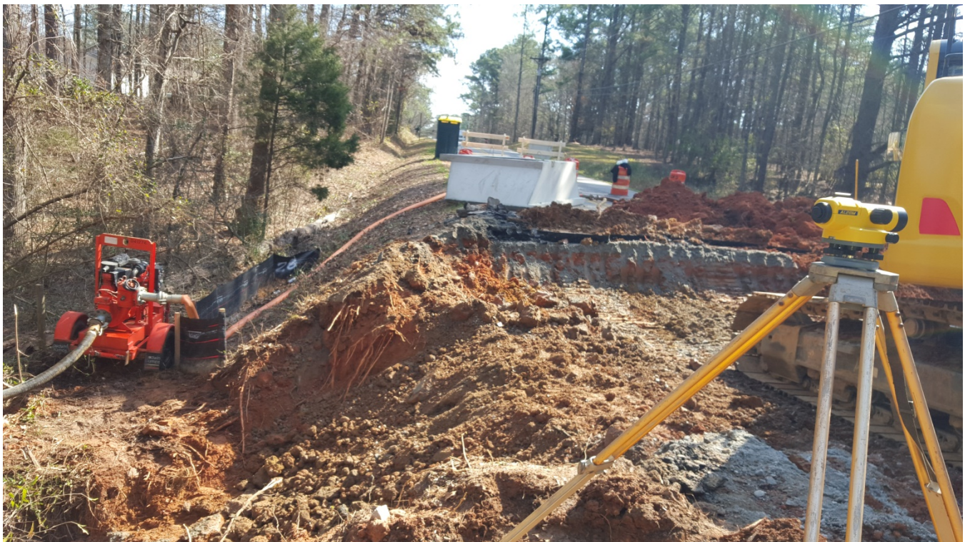
Photo 2: Water was pumped around the project site to allow for dry installation of new pipe.
