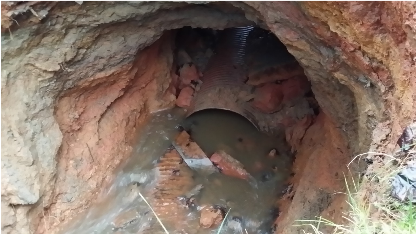
Photo 1: Pre-existing condition of 54" metal pipe. Washout, during the December 2015 rain event, occurred around the pipe resulting in complete road failure.
