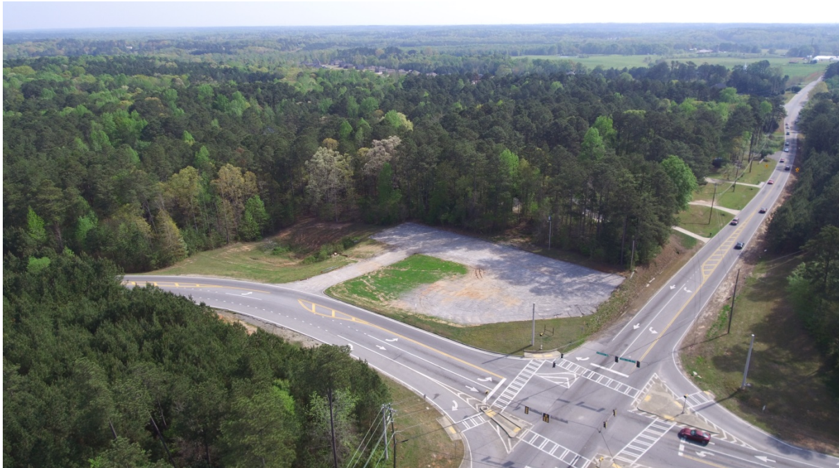
Photo: Ariel photo of future site location of Fire Station 4.
