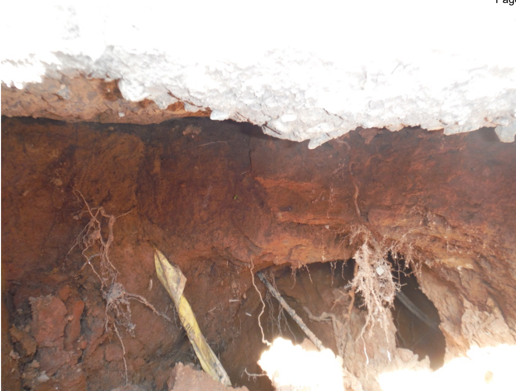
Photo 1: Sink hole caused by pipe.
