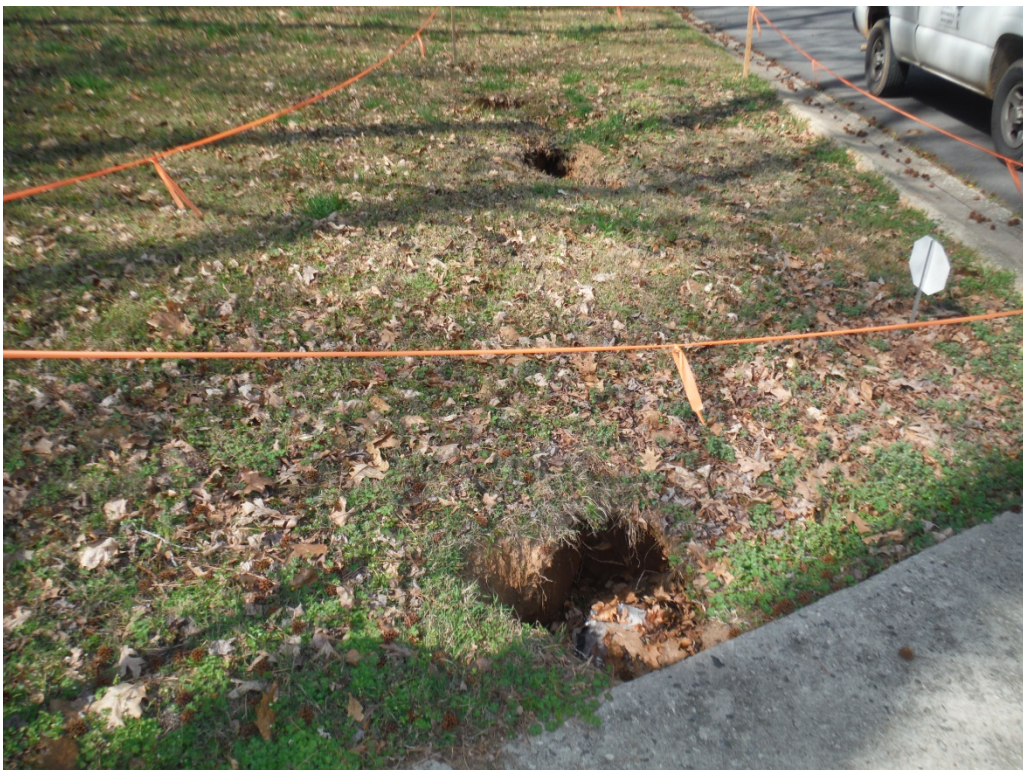
Photo 2: Sink holes caused by failing pipe system.
