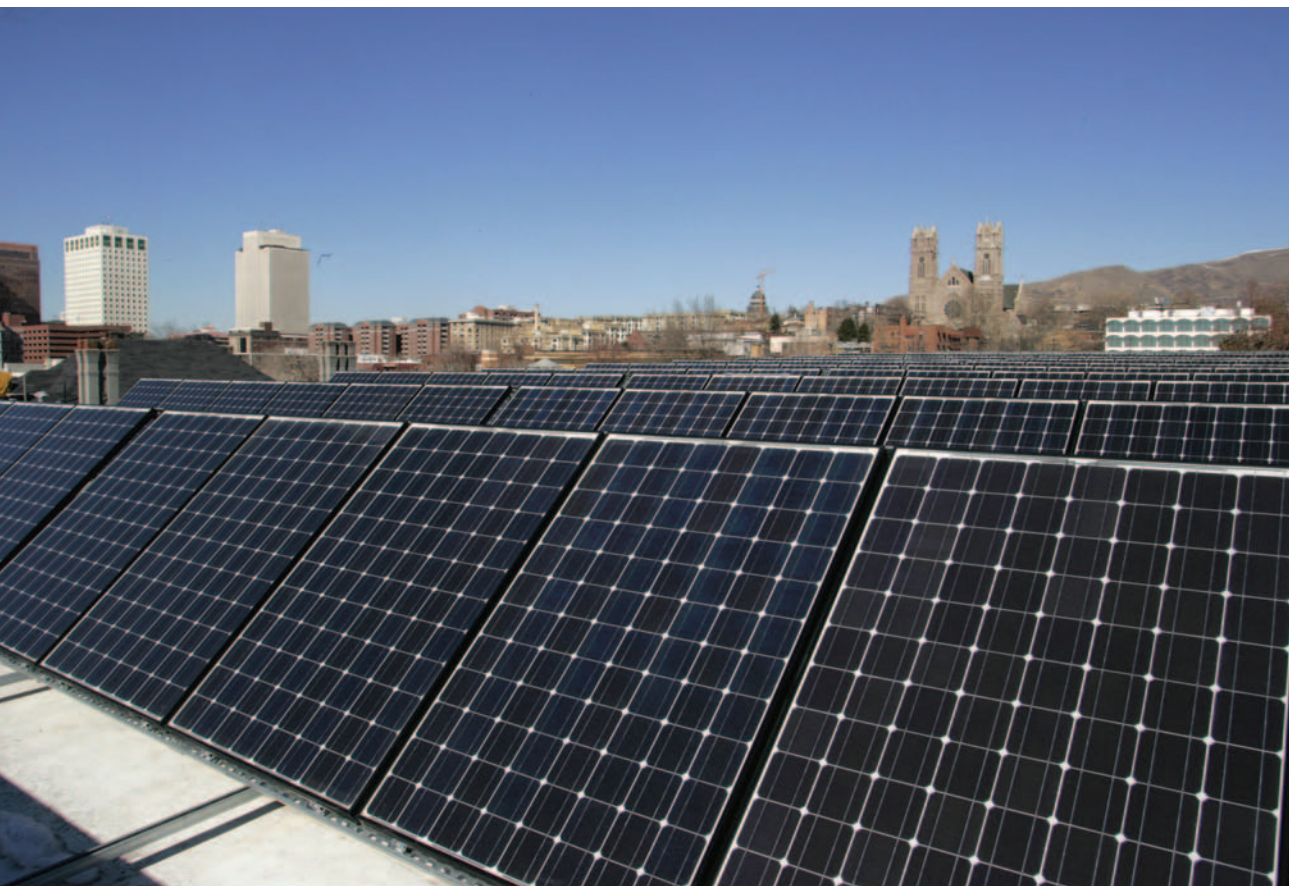
A 25-kW solar PV system provides power to the county-owned Clarke Planetarium in downtown Salt Lake City. (SLC/PIX18364)
