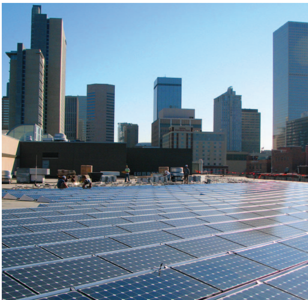
Namaste Solar was responsible for this 300 kw PV rooftop installation on top of the Colorado Convention Center in Denver, Colorado. (Namaste Solar Electric/PIX18044)
