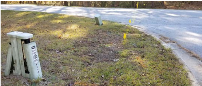
L Marked Gas-line (AGL) & AT&T Telephone Pedestal
