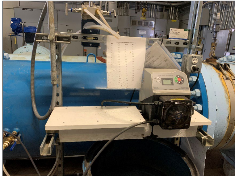
Figure 12. Permanganate Injection at Lake Horton Raw Water Pump Station
