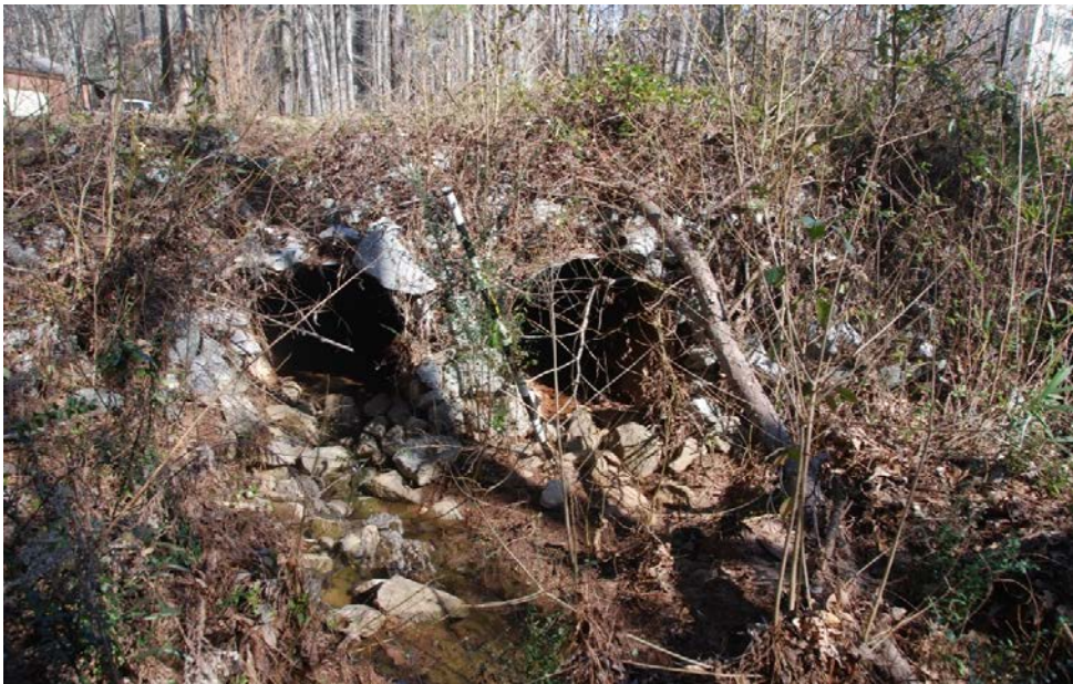
Photo 2: Downstream end of culverts
