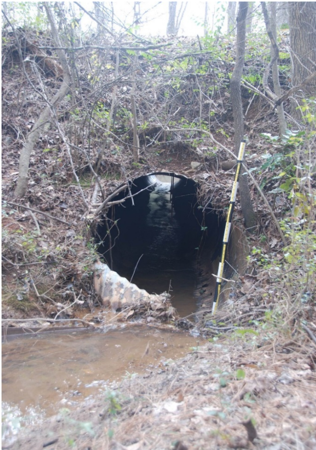
Photo 1: Upstream end of culvert.
