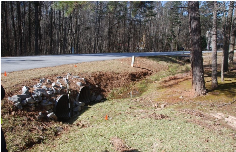
Photo 1: Upstream end of culverts looking southwest towards Angela Dr.
