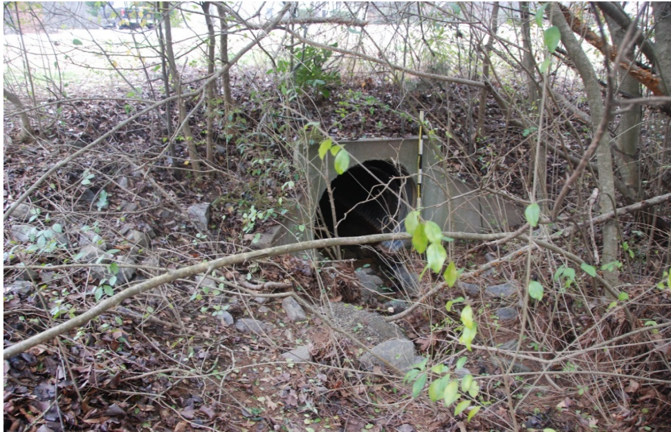
Photo 1: Upstream end of culvert
