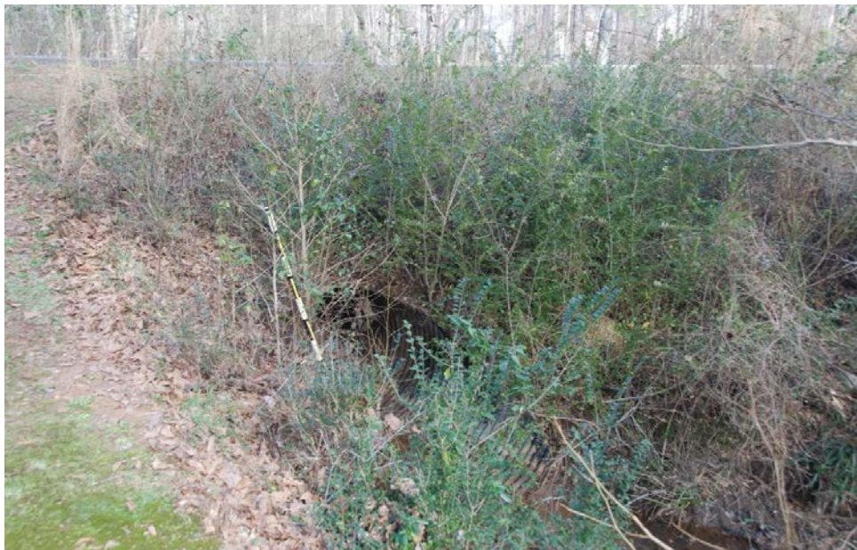
Photo 2: Downstream end of culvert looking northeast towards Branchwood Ct.
