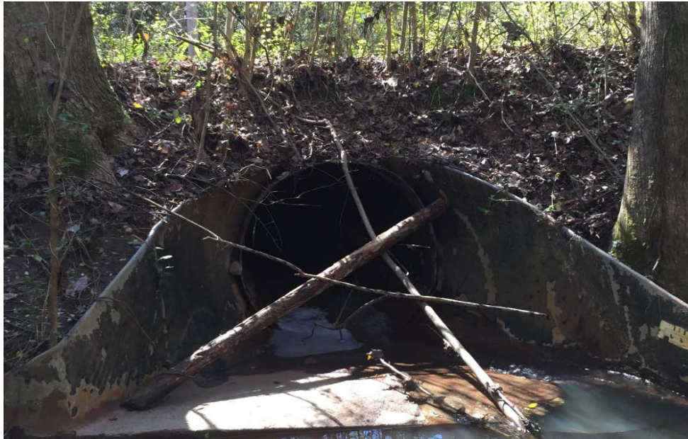
Photo 1: Upstream end of culvert looking South towards North Bend Court
