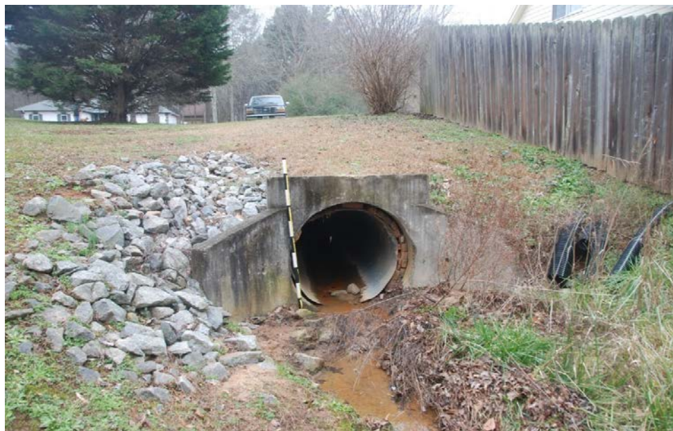
Photo 2: Downstream end looking East towards Ridge Brook Court
