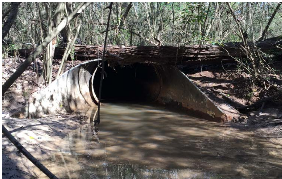
Photo 2: Downstream looking South towards North Bend Court.
