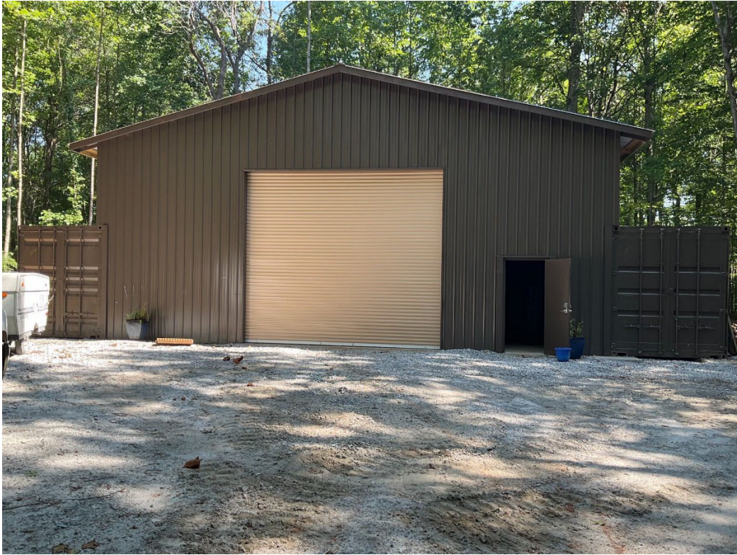
UNPERMITTED STRUCTURE (BUILDING SAFETY)
