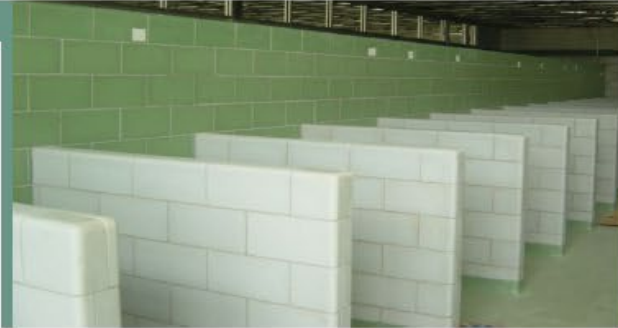
Interior Kennel Space Material - GLAZED CMU New kennels could be constructed using glazed CMU, which is easier to clean, resulting in a more hygienic space.
