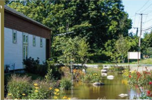
Bioretention - After Rain Event Water retention with planting.
