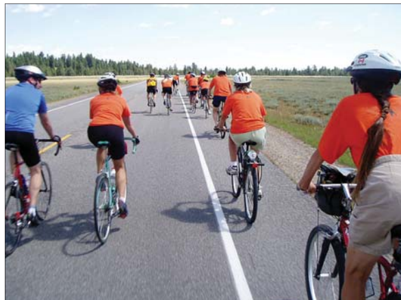
Roadway rehabilitation can include shoulder width to accommodate bicycles. This is typically no wider than recommended vehicle-based design for these shoulders.
