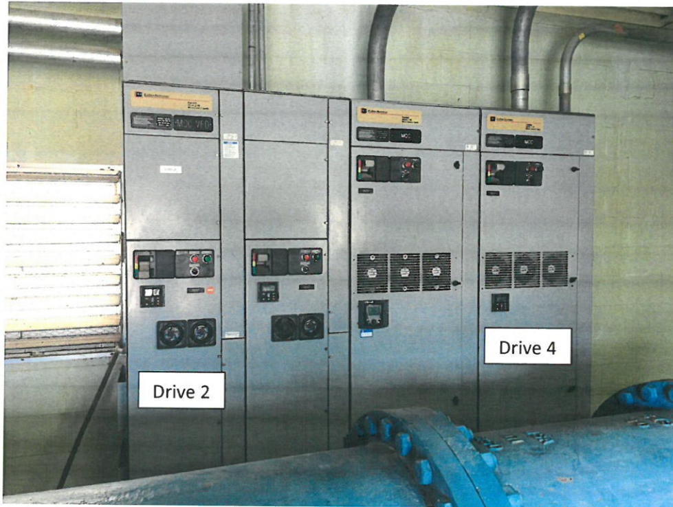
Figure 3 - RWPS MCC Drive Cabinets
