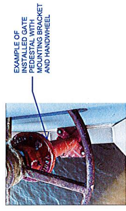
EXISTING GATE OPERATOR ON EAST FACE OF BUILDING
