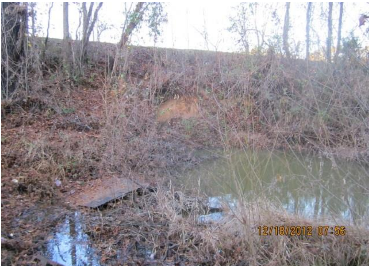
2012 PHOTO: VIEW OF DOWNSTREAM AREA WHERE THE PSP DISCHARGES. THE DOWNSTREAM END OF THE PIPE IS SUBMERGED.
