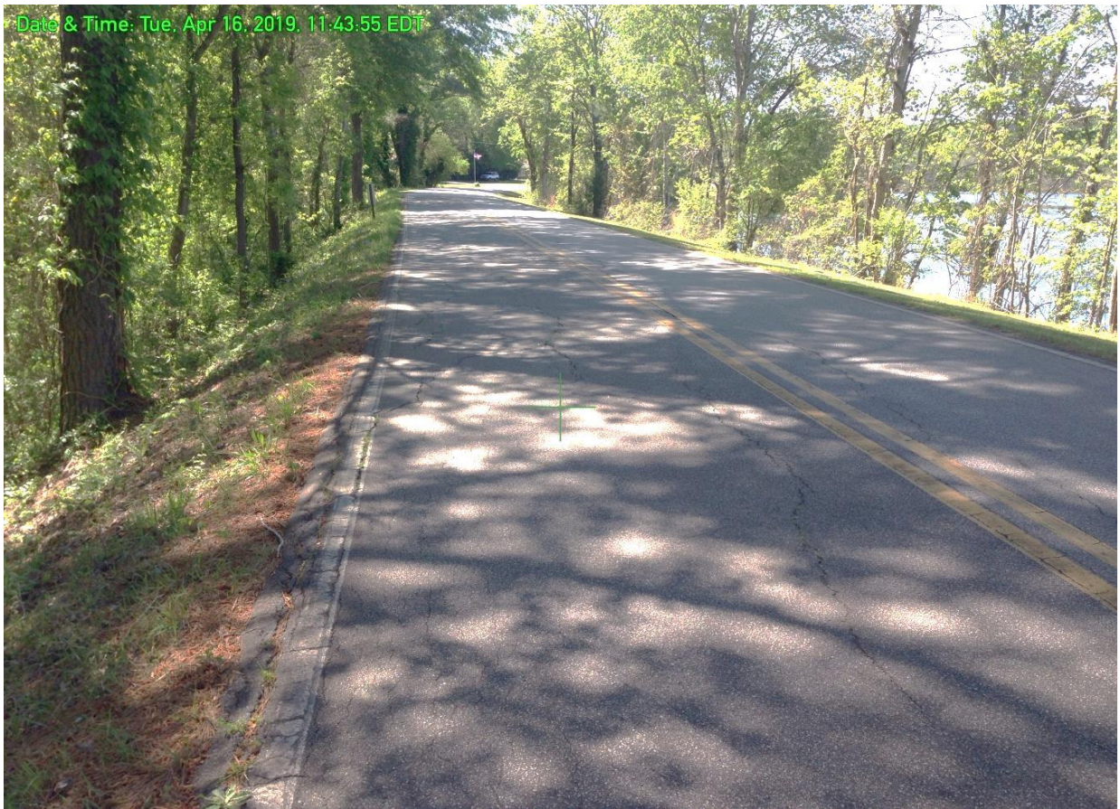
VIEW LOOKING SOUTH ALONG THE DOWNSTREAM SLOPE FROM ABOUT MIDWAY OF THE DAM.
