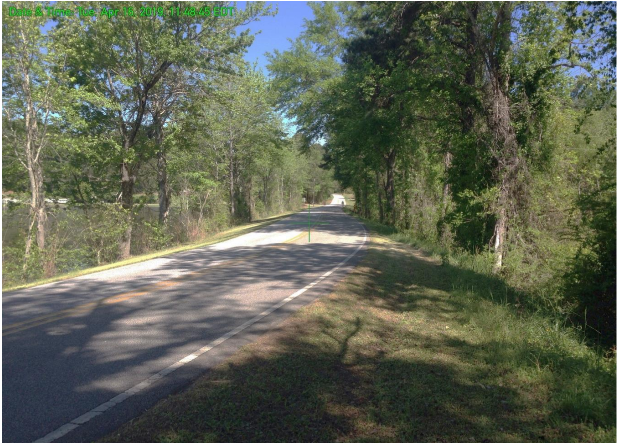
VIEW LOOKING NORTH ALONG LONGVIEW ROAD FROM NEAR SOUTH END OF DAM.
