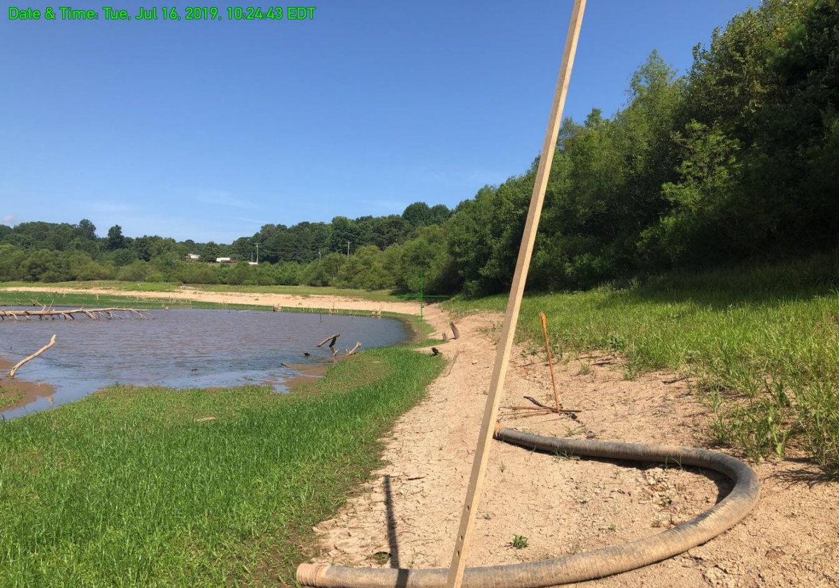
VIEW LOOKING LEFT ALONG UPSTREAM SHORELINE FROM NEAR LOW LEVEL PIPE WITH LAKE ESSENTIALLY DRAINED. REMNANTS OF OLD PVC AND RUBBER PUMP PIPE PRESENT IN THIS AREA.
