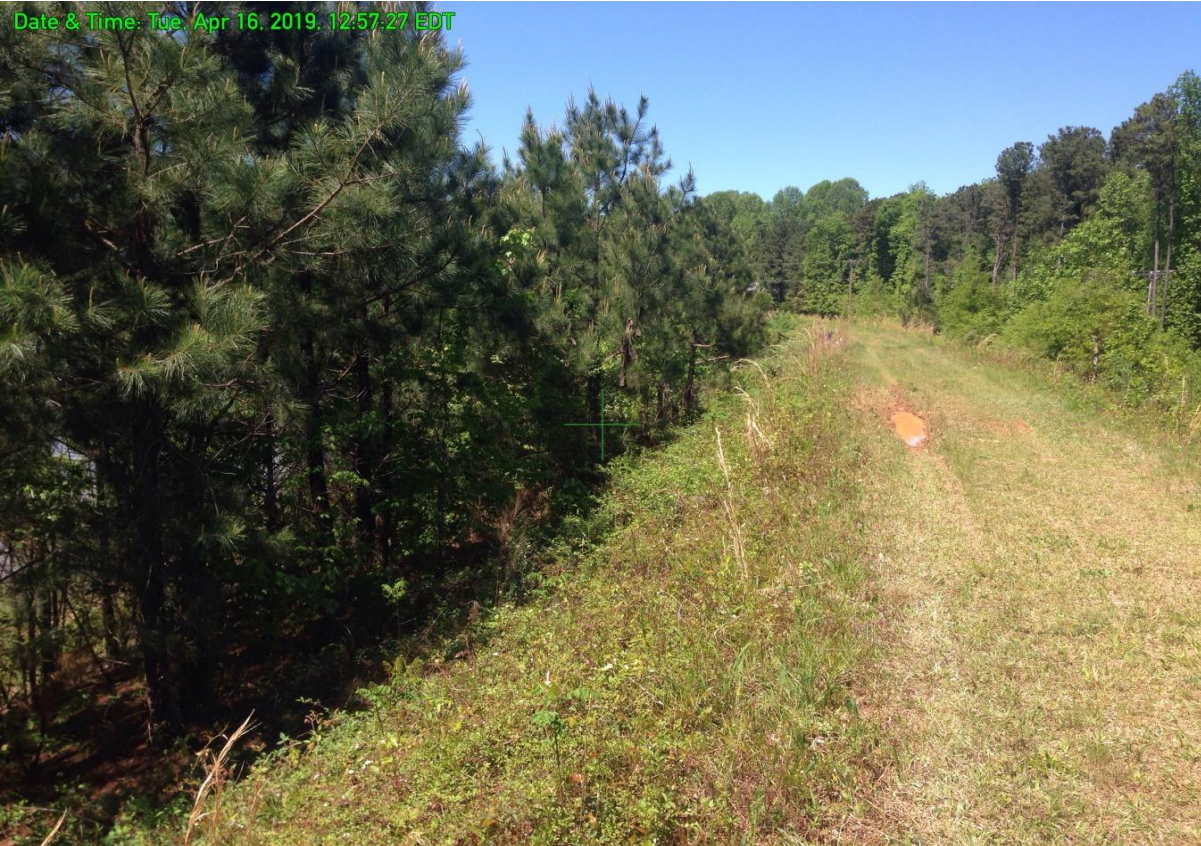
VIEW ALONG THE DAM CREST FROM NEAR THE RIGHT END.
