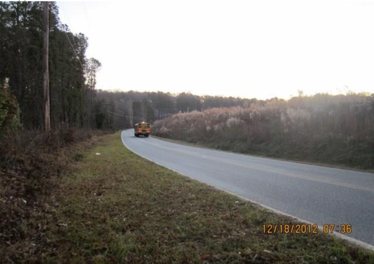
2012 VIEW LOOKING LEFT TO RIGHT ALONG NEELY ROAD FROM NEAR LEFT END OF DAM.
