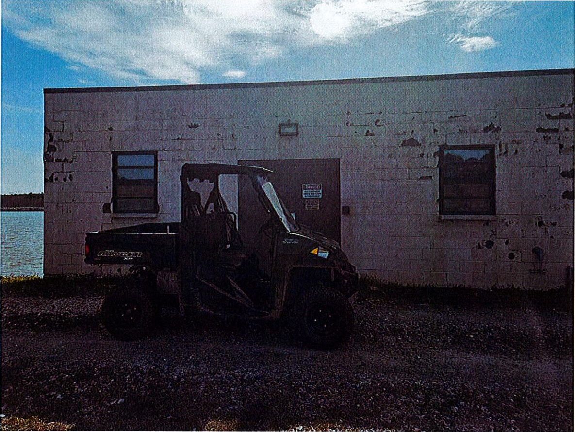
Crosstown WTP Raw Pump Building
