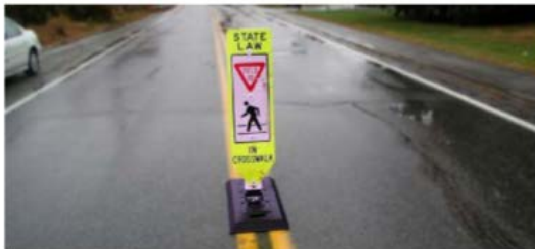
Image 16: In-Street Pedestrian Crossing Sign
