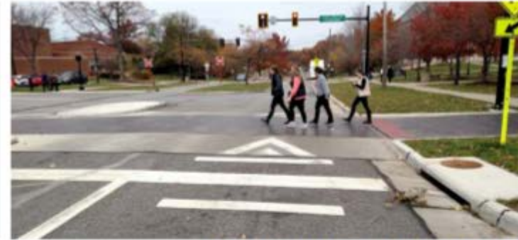
Image 12: Raised Crosswalk, University Heights
