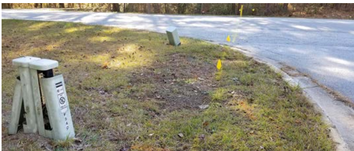
L Marked Gas-line (AGL) & AT&T Telephone Pedestal
